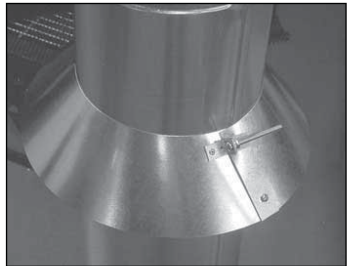
Figure 10.17 Assembling the Storm Collar Around the Pipe
